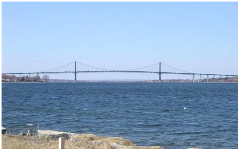
Mount Hope Bridge – 1927 Bristol to Portsmouth, RI Main span of 1200 feet Construction cost of $2.5 million
